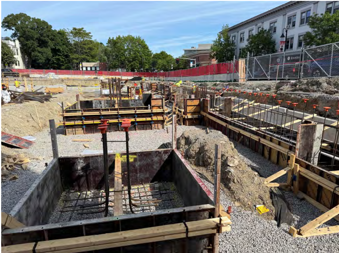
Forms and rebar along 1/1.3/2 lines
