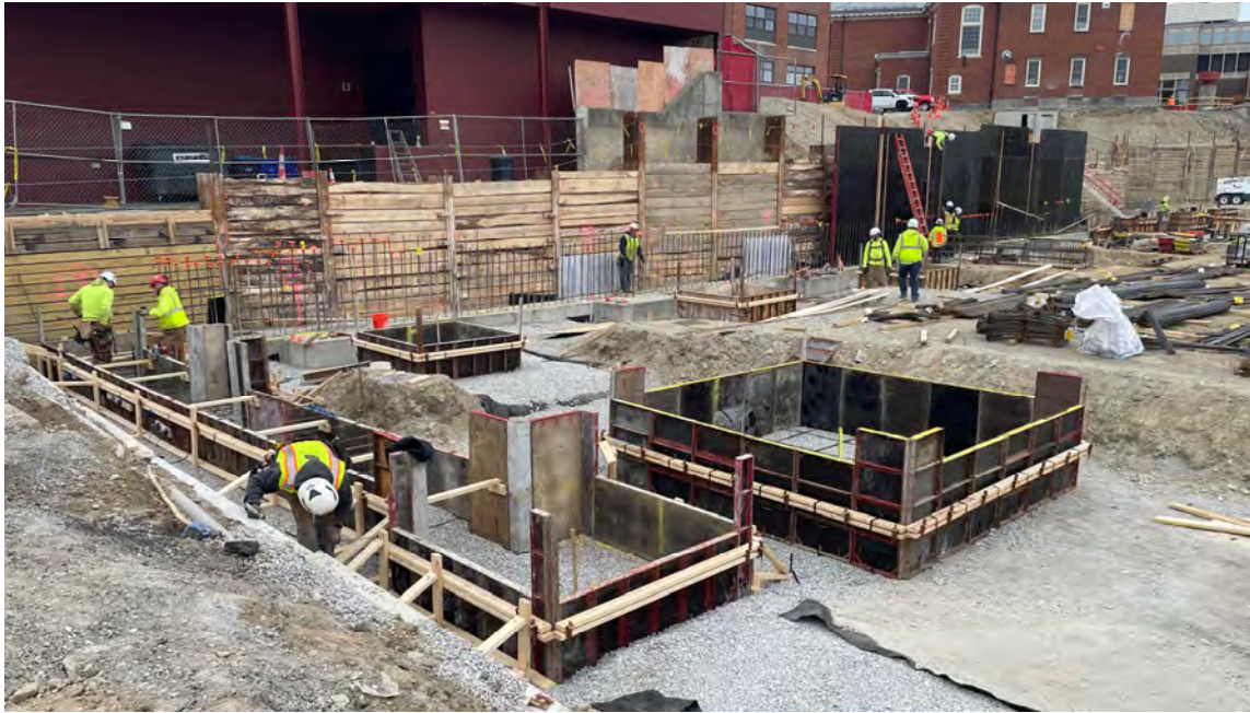
Forms and rebar turn the corner on Harvard Street (1/1.3/2 lines)
