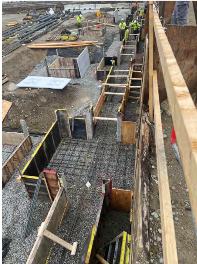
Footing forms and rebar, 'A' line
